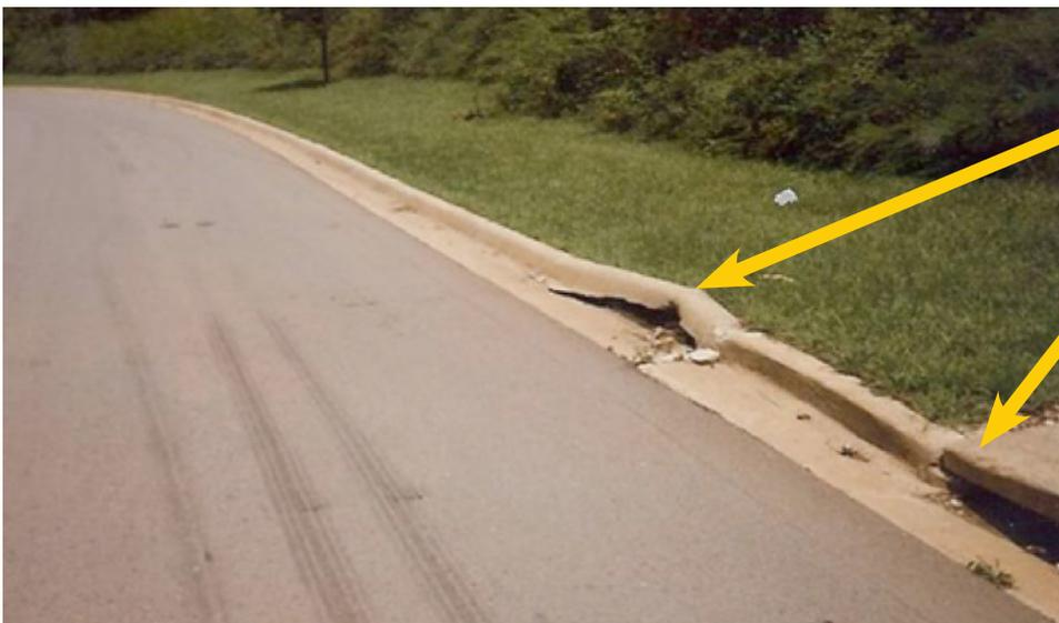
Figure 3. Blow-ups can also occur in curbing.
