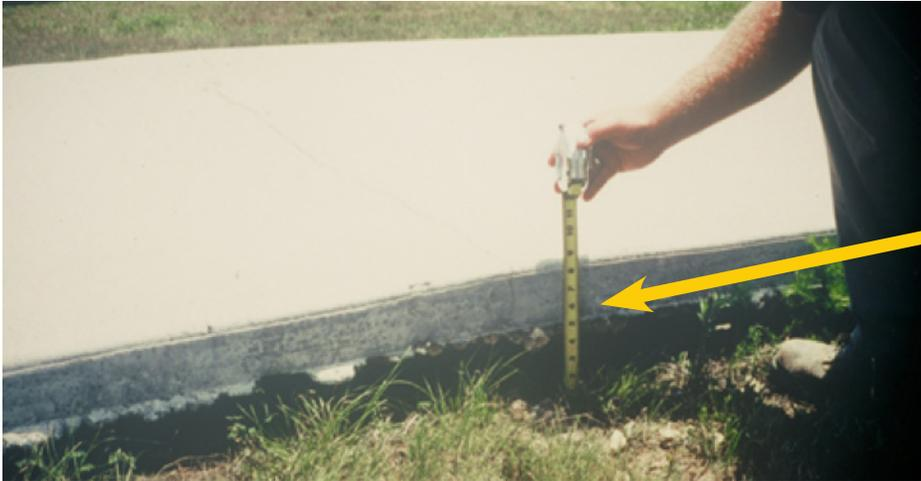
Figure 1. This slab has "blown up" about 5"
