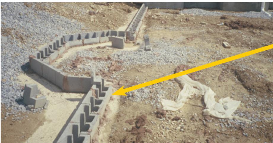
CMU form-blocks are popular methods of forming up a slab, but they lock the slab concrete into the CMU which is already bonded to the footing. This restricts slab movement.
