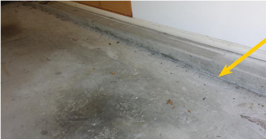
Concrete slab placed directly against the stem-wall foundation. No isolation joint material. Resulting in the slab bonding to the wall; restraining slab movement and no allowance for differential movement between the slab and the wall.
